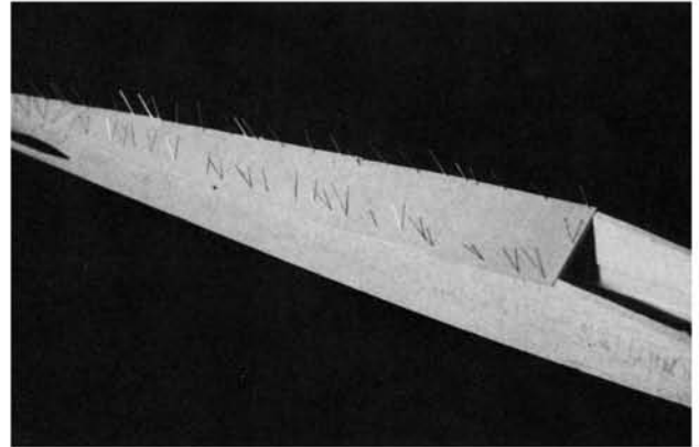
Installing 1/8" bottom sheeting (cross grain).
